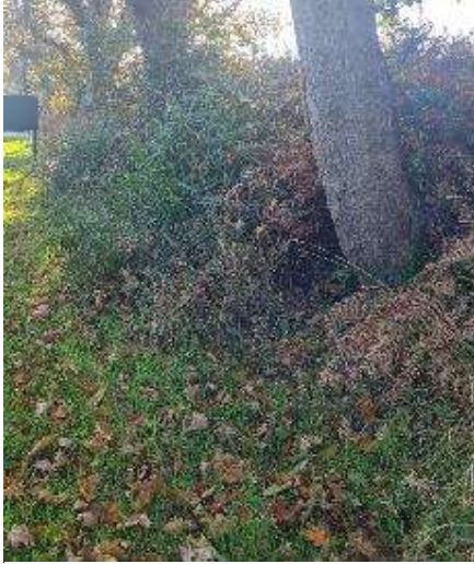
Photo 1: Northern limit of drainage ditch, looking south
